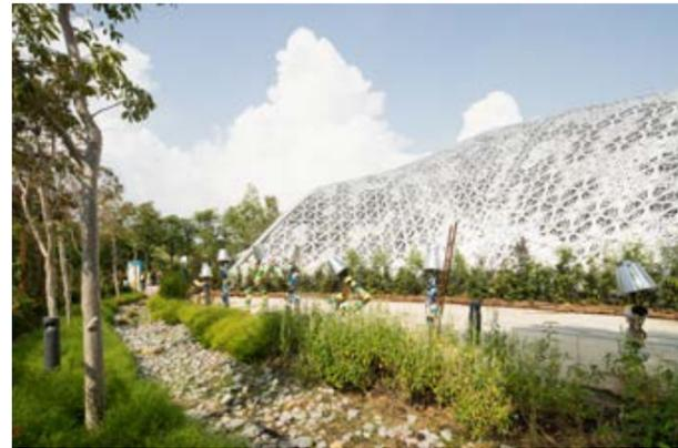
The light-filtering effect of the project is based on about 11,000 triangular aluminium panels of differing perforations
